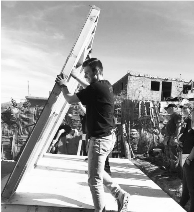
Lifting the first wall. Photo Credit: Dr. Cliff Pawley
